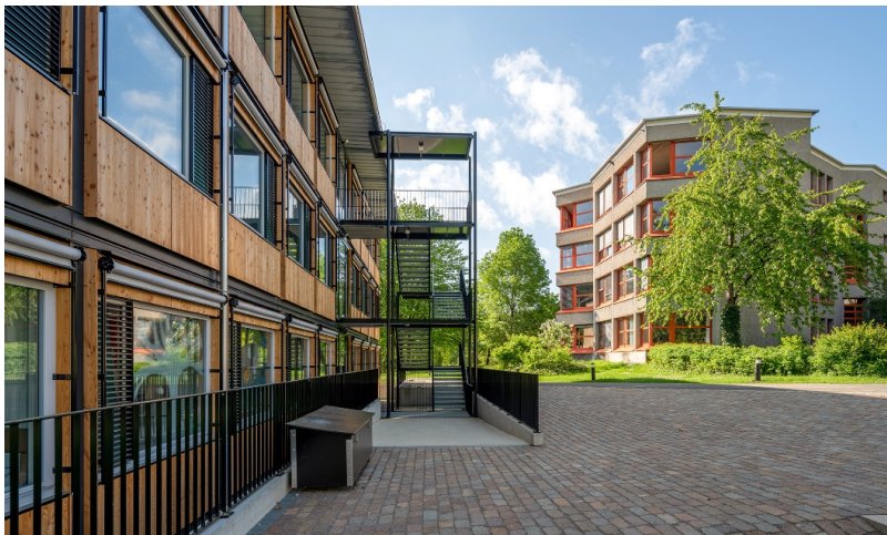
The school pavilion's different levels are accessed via an external staircase.
