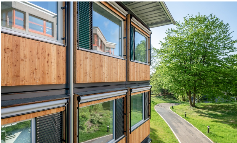
Timber facade of the modular school pavilion
