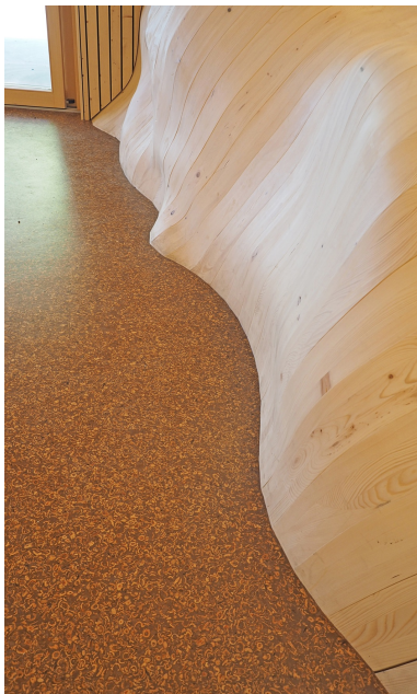
When combined, the individually shaped components produce the curves typically found on a walnut.
