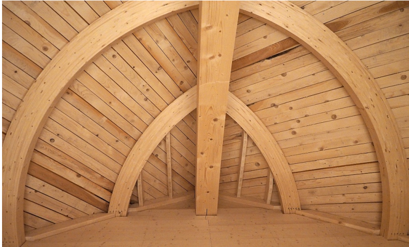
Looking at the roof cladding's supporting structure from the inside.
