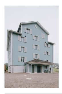
The facade consists of eternit shingles, in keeping with the parameters of the townscape.
