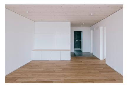
The wooden floor and exposed woodconcrete composite ceilings create a cosy indoor atmosphere.
