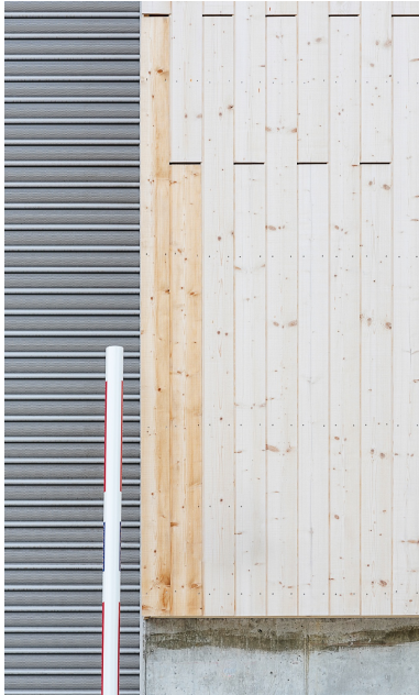
The UVood-treated facade compared side by side with several natural facade boards.
