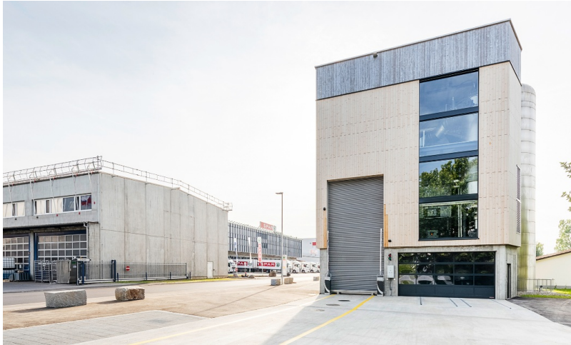
The energy plant with timber facade in two different treatments.
