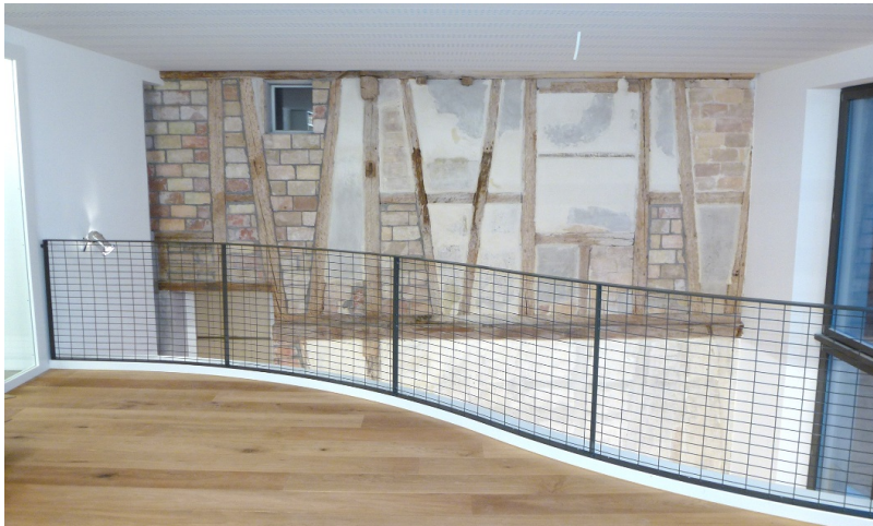
Renovating the old masonry
