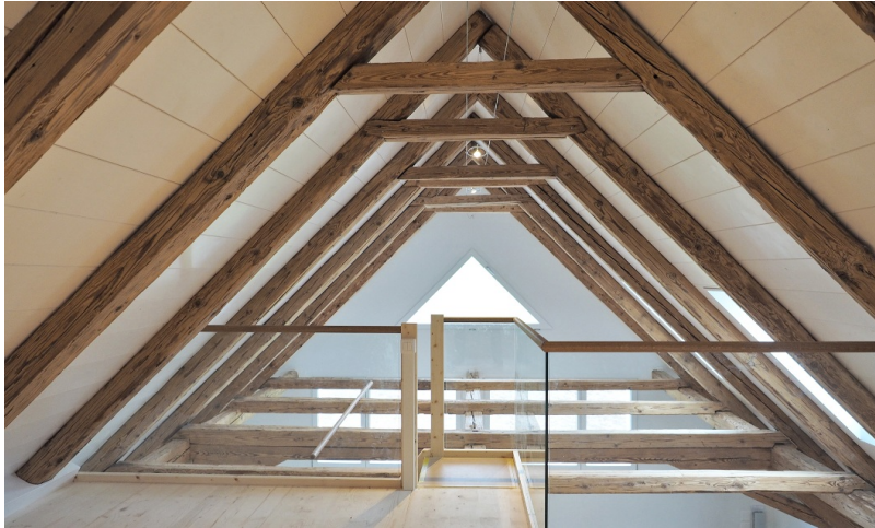
Roof truss, renovated and remodelled
