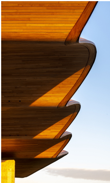
Impressive roof construction in oak
