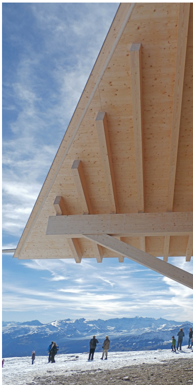
Close-up of the roof construction
