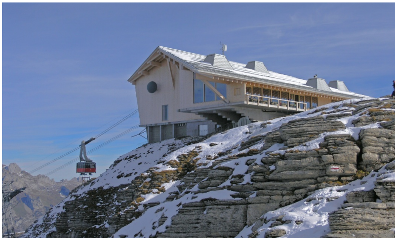
South-west view of the mountain restaurant
