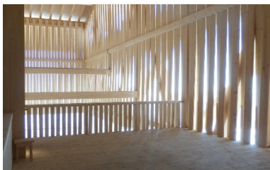
Close-up of the timber construction
