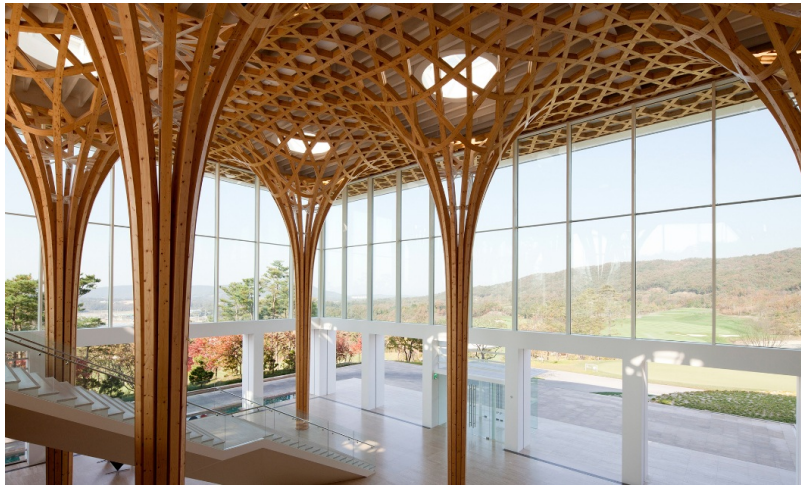
View of the fascinating vaulted roof
