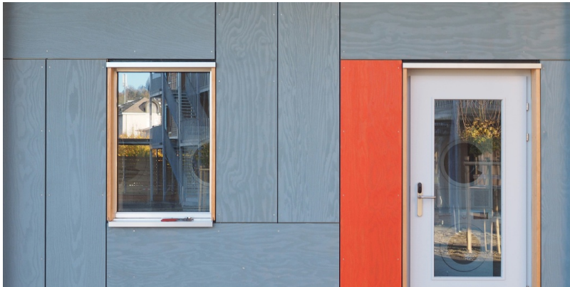
Close-up of the facade in grey and red
