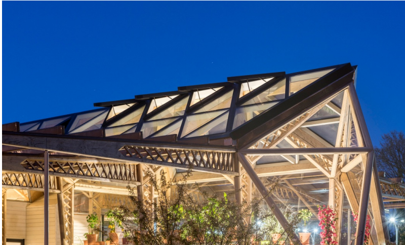
Timber roof construction
