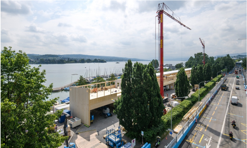
Building a temporary pit lane
