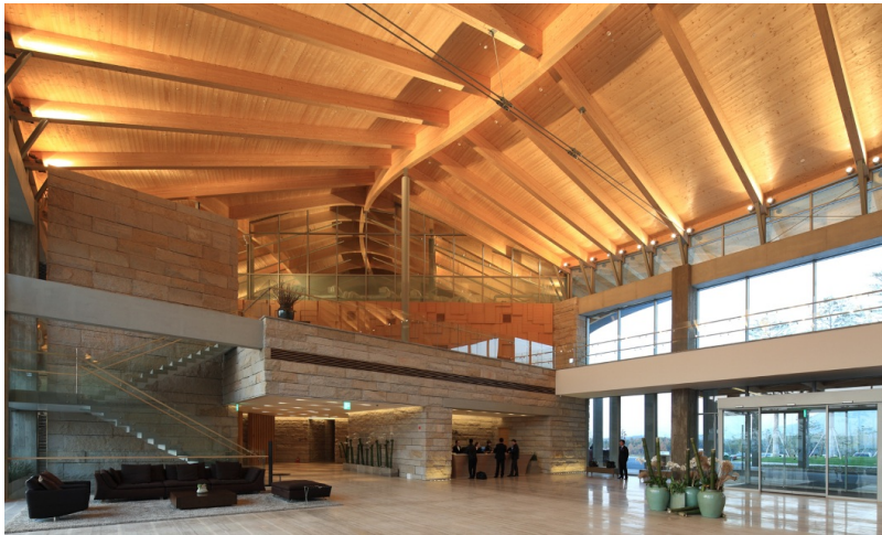
Sweeping, leaf-shaped roof construction
