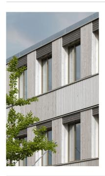
The exterior design of the four-storey modular building is characterised by a timber façade consisting of pre-greyed, vertically and openly laid spruce/fir strips and horizontal rhomboid profiles.
