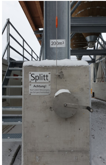
Hot-dip galvanised roof platform
