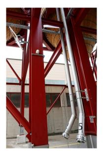
Filling pipes for the salt
