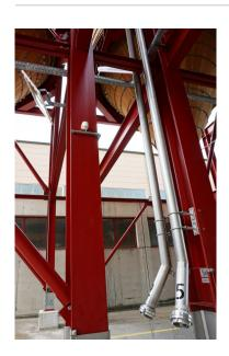
Filling pipes for the salt
