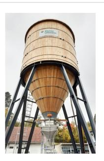
Access ladder with hot-dip galvanised steel
