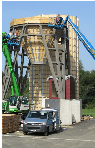
Loading by belt weigher at the silo hopper at the gritting silo facility
