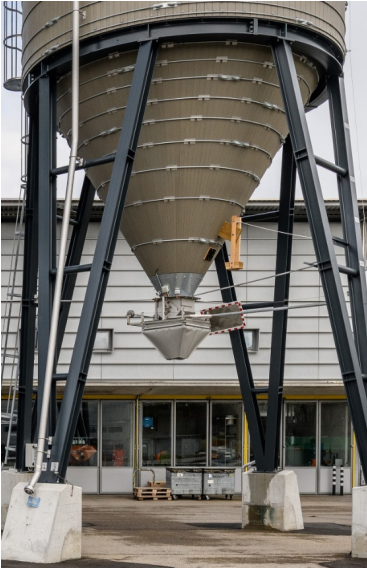
Round wooden silos with a capacity for salt of 200m 3 each
