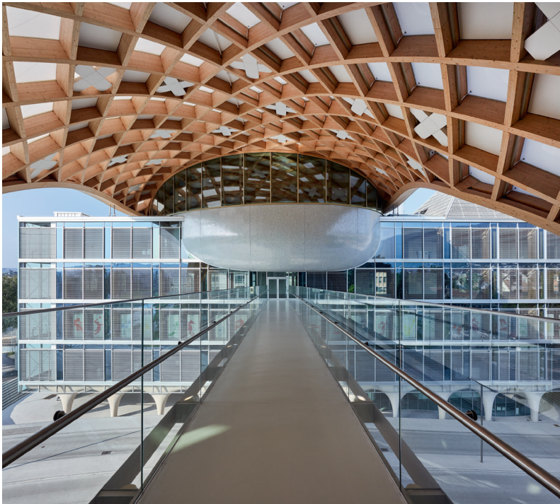
The elongated Swatch headquarters is covered with a giant timber-lattice supporting structure.
