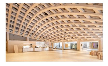
The unsupported Free Form roof made of laminated veneer lumber and arranged as a visible lattice shell spans an area of 25 x 48 metres.
