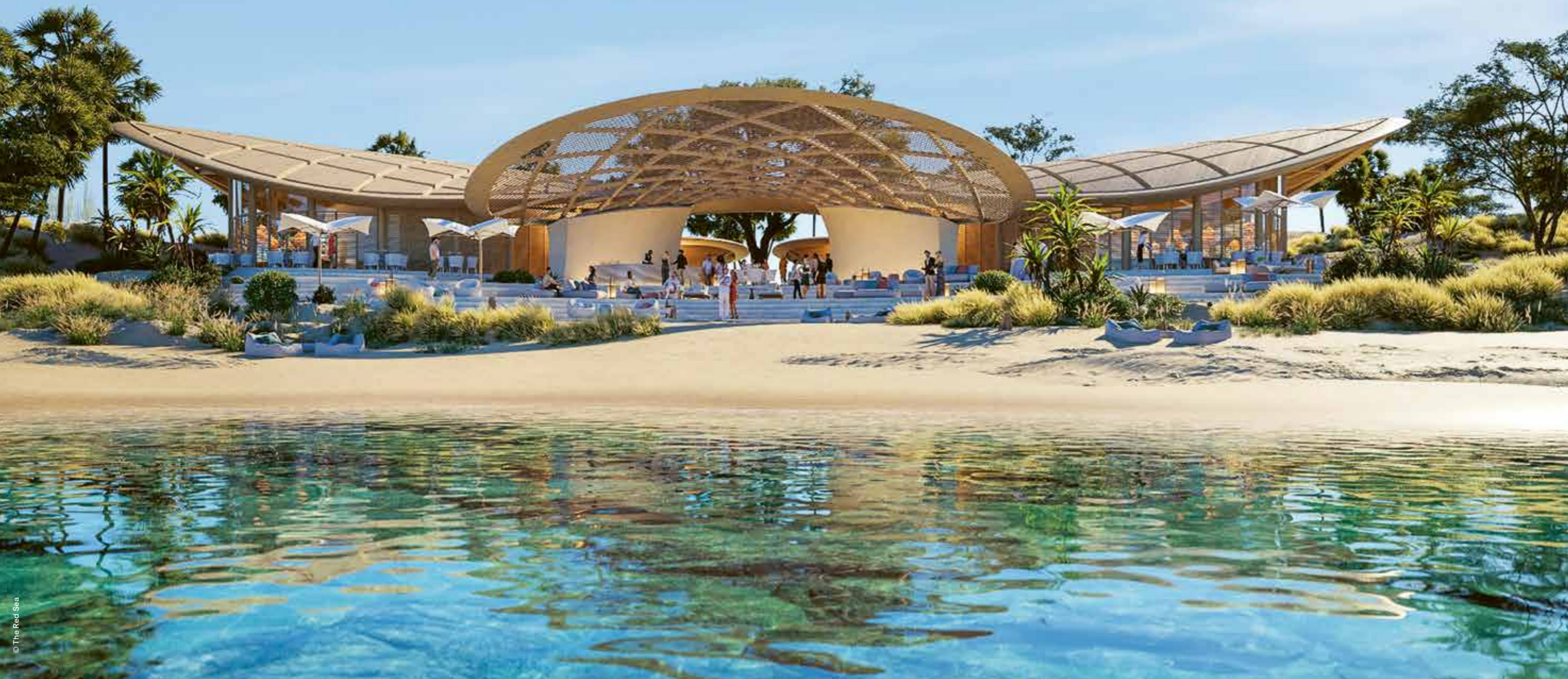
One of the luxury buildings forming part of the new tourist destination 'The Red Sea' is the golf clubhouse with its Free Form roof on Shura Island.
