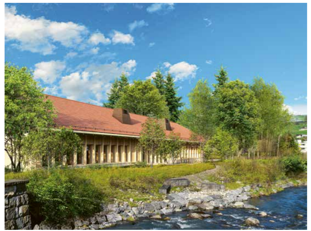
↑ The spruce wood used for the interiors of the seminar rooms creates a positive indoor climate. ← The new seminar building is in an idyllic location on a strip of land where two rivers meet. → The star-shaped bathing and sauna building has virtually no external walls and is clad in plenty of glass.
