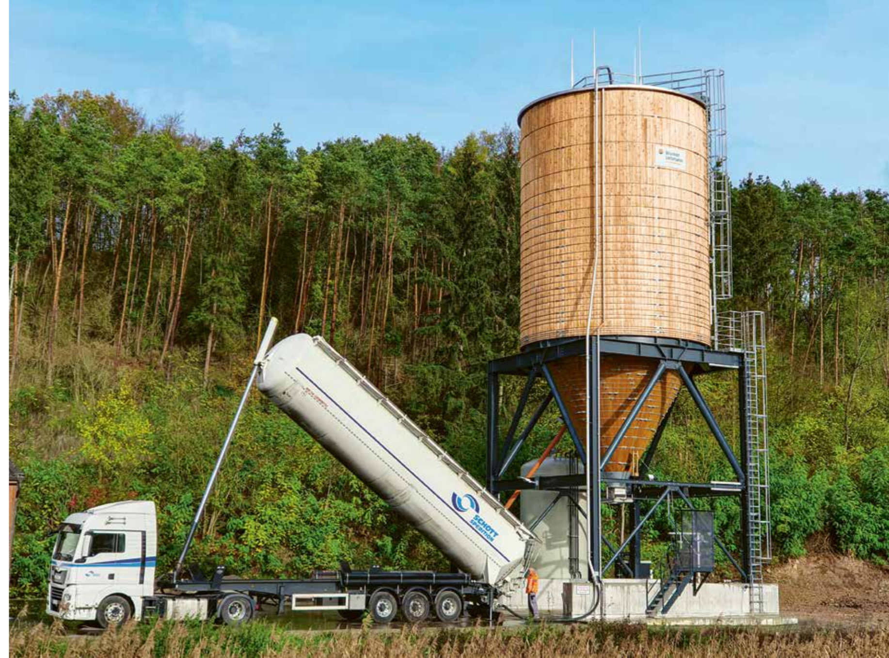
Filling the silo with rock salt via the filling pipe.
