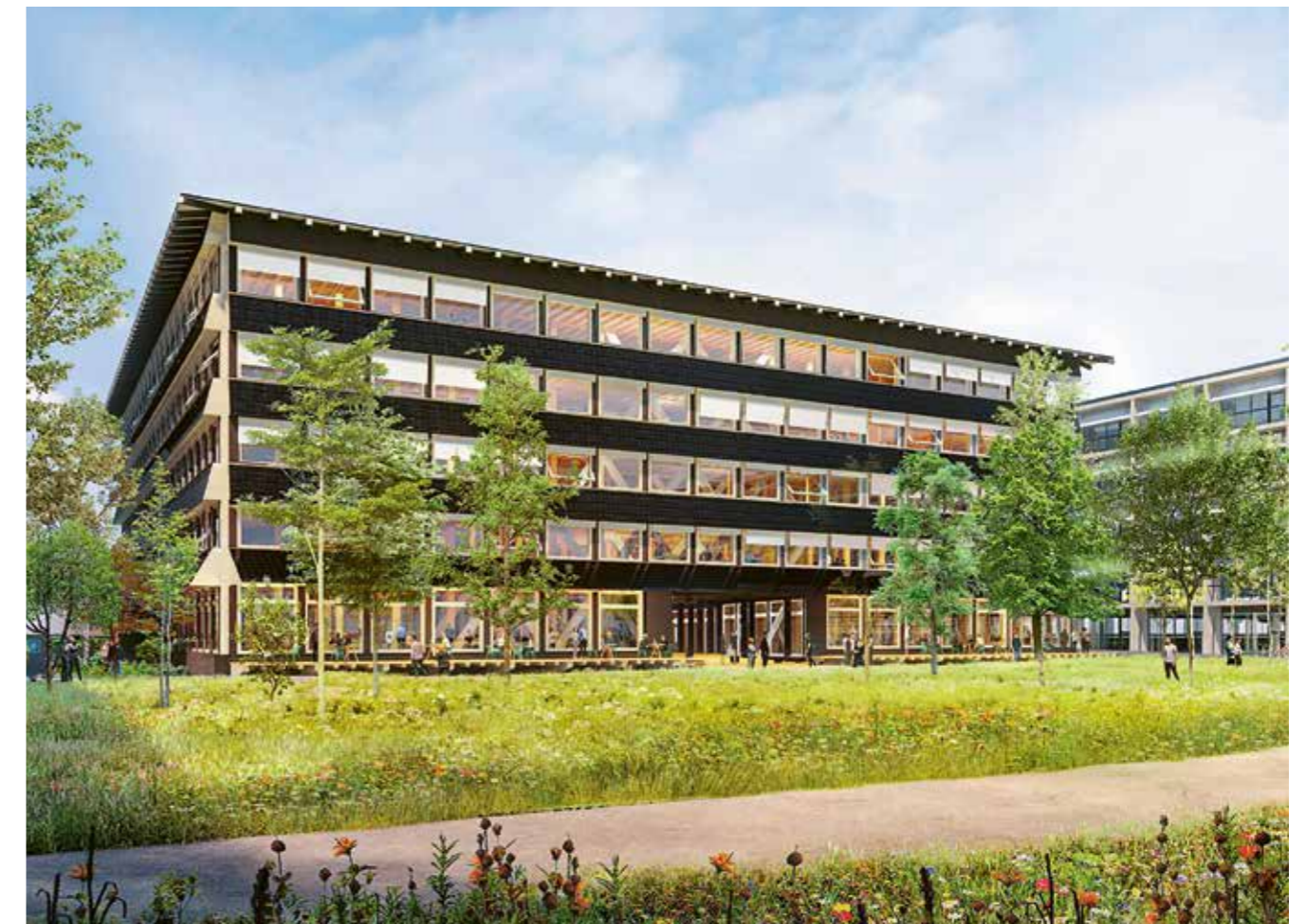
↶ A full-storey mock-up helped to resolve structural questions and material choices early on. ← HORTUS sets new standards for sustainable construction with components made from natural materials subject to circular processing.
