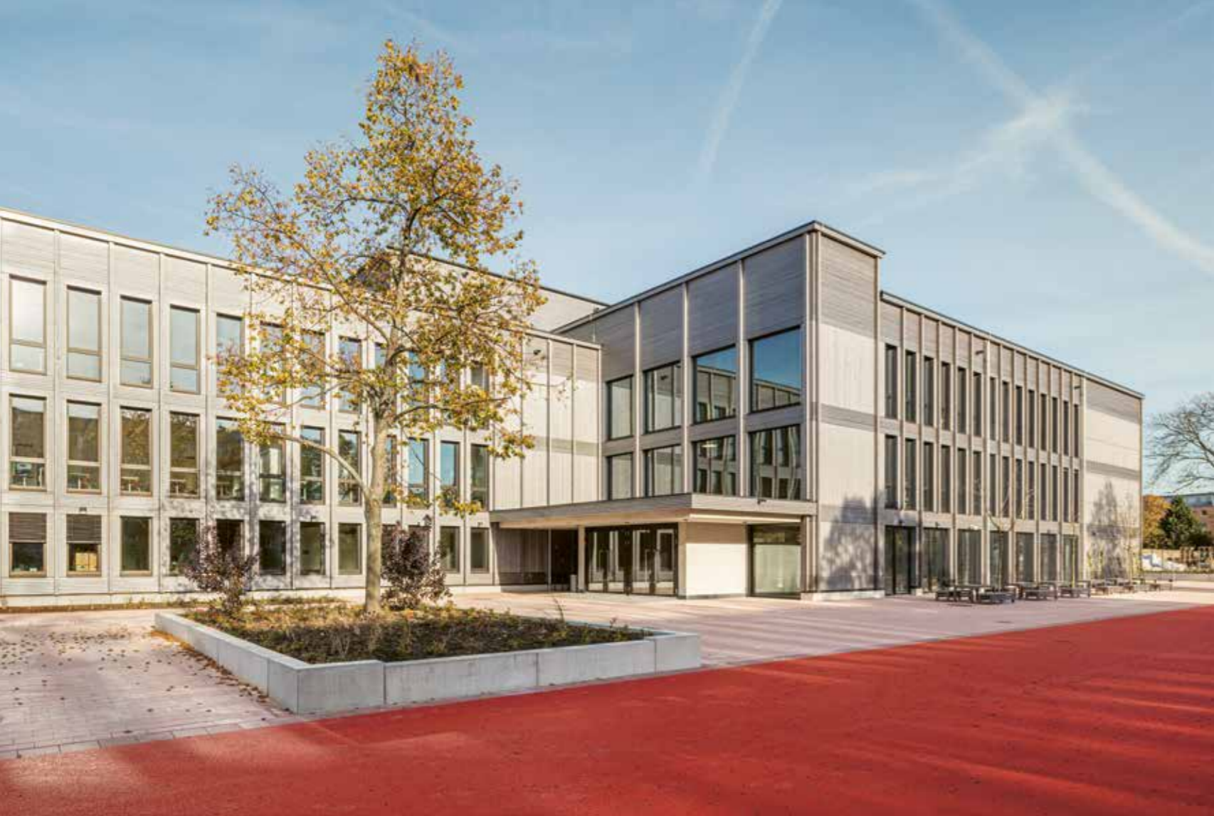
The three-storey school building in a hybrid timber modular/element construction features 28 classrooms, a kitchen and a canteen.
