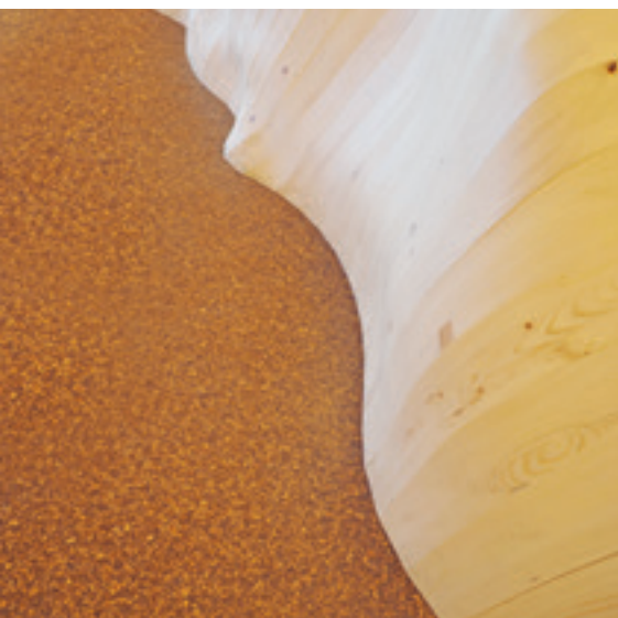
Local nutshells are worked into the specially made flooring, GIOMOFLEX® naturo by Uniquefloor.
