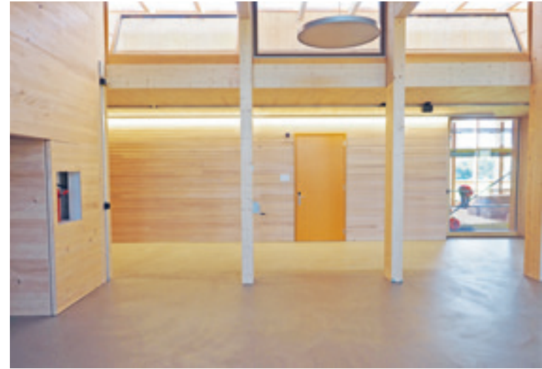
The cross-ventilation is a key element in ensuring comfort.
